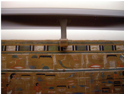
Fig. 11. A detail of the new clips that hold the upper edge of the panel, after final adjustment and painting.
