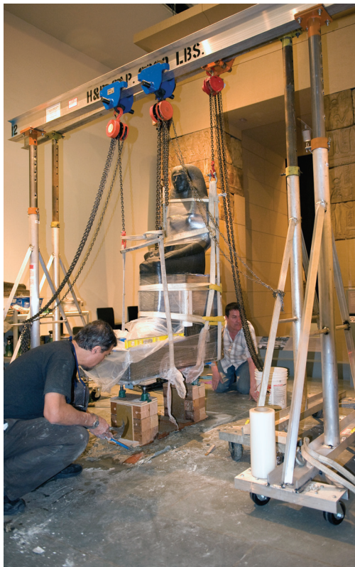
Fig. 19. The concrete base has been removed, and the sculpture remains supported by the temporary support system. The gantry continues to provide additional security during this transitional moment before installation of the steel armature. © 2011 Museum of Fine Arts, Boston.
